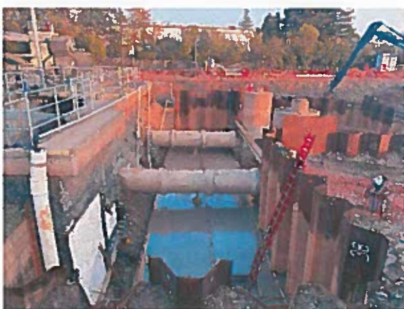
Wet well area excavated, and dewatering wells installed.
