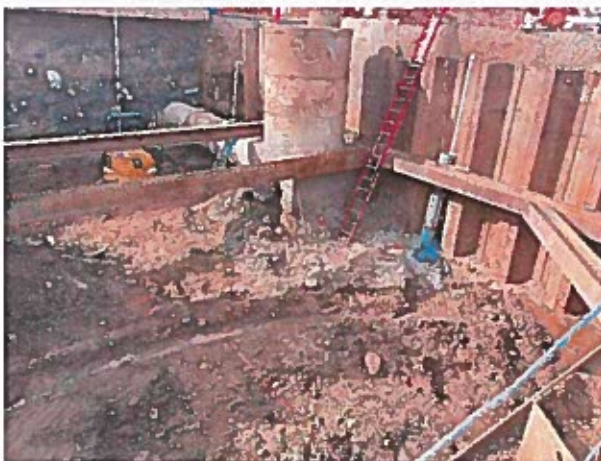
Wet well area excavated, and dewatering wells installed.
