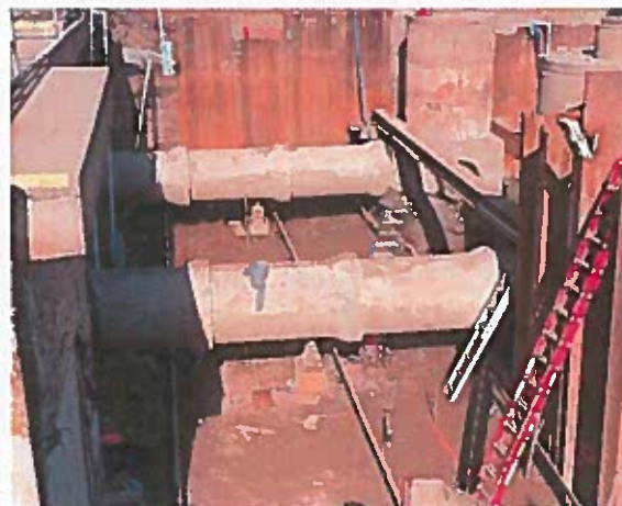
Influent vault area leveled, and formwork was installed for rat slurry slab pour.
